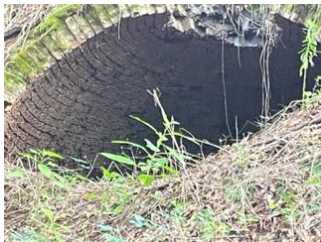
Blocton Coke Oven Close Up
