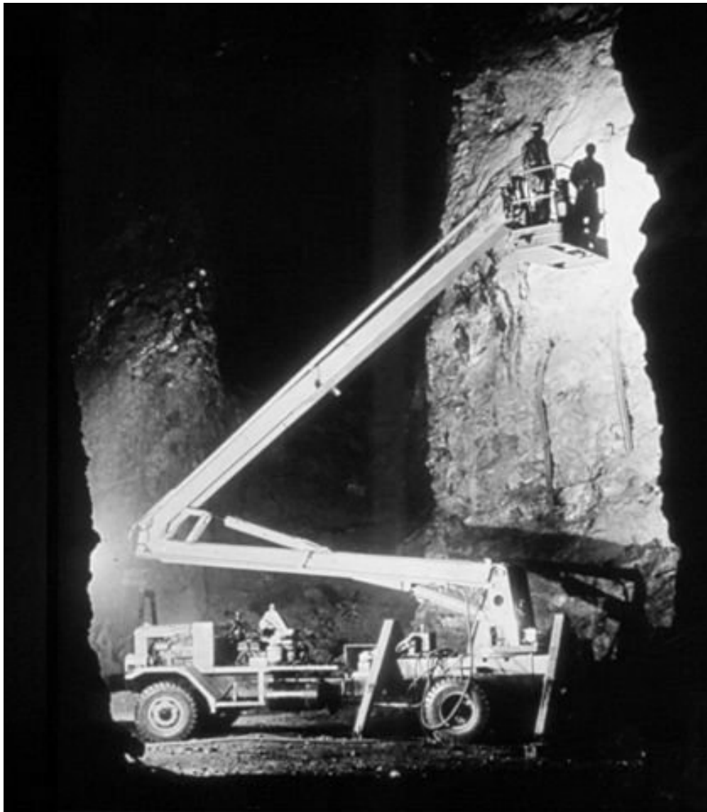
Scaling loose rock in the Friedensville Mine, ca. 1976. (Courtesy of Ken Cox.)
