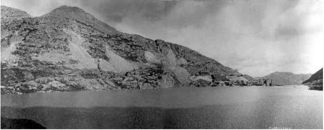
The Iowa Mine on the left, the Silver Lake Mine on the right, with Round Mountain in the background, taken around 1900 from the Royal Tiger Mine on the east bank of Silver Lake. (Courtesy of the San Juan County Historical Society, J-2-C-5-20-a.)
