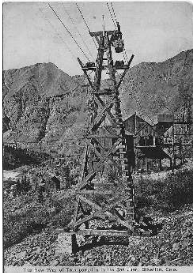
This postcard view shows the Bleichert tramway that descended from the Iowa Mine on Silver Lake to its mill in Arrastra Gulch. Note the man riding in a bucket. (Courtesy of the Denver Public Library, Western History Collection, X-62249.)
