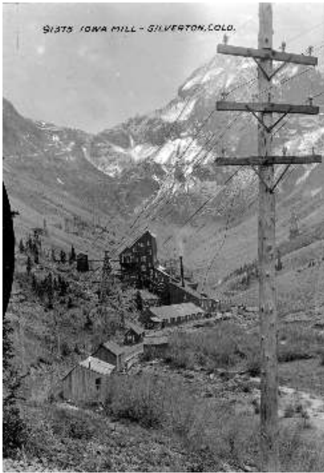
South view of the frame Iowa Stamp Mill, Arrastra Gulch, 1902. The gulch's headwall, beyond which lies Silver Lake, appears at the top. Note the telegraph poles and the towers of the multitude of tramway systems. (Courtesy of the Denver Public Library, Western History Collection, Z-2560.)
