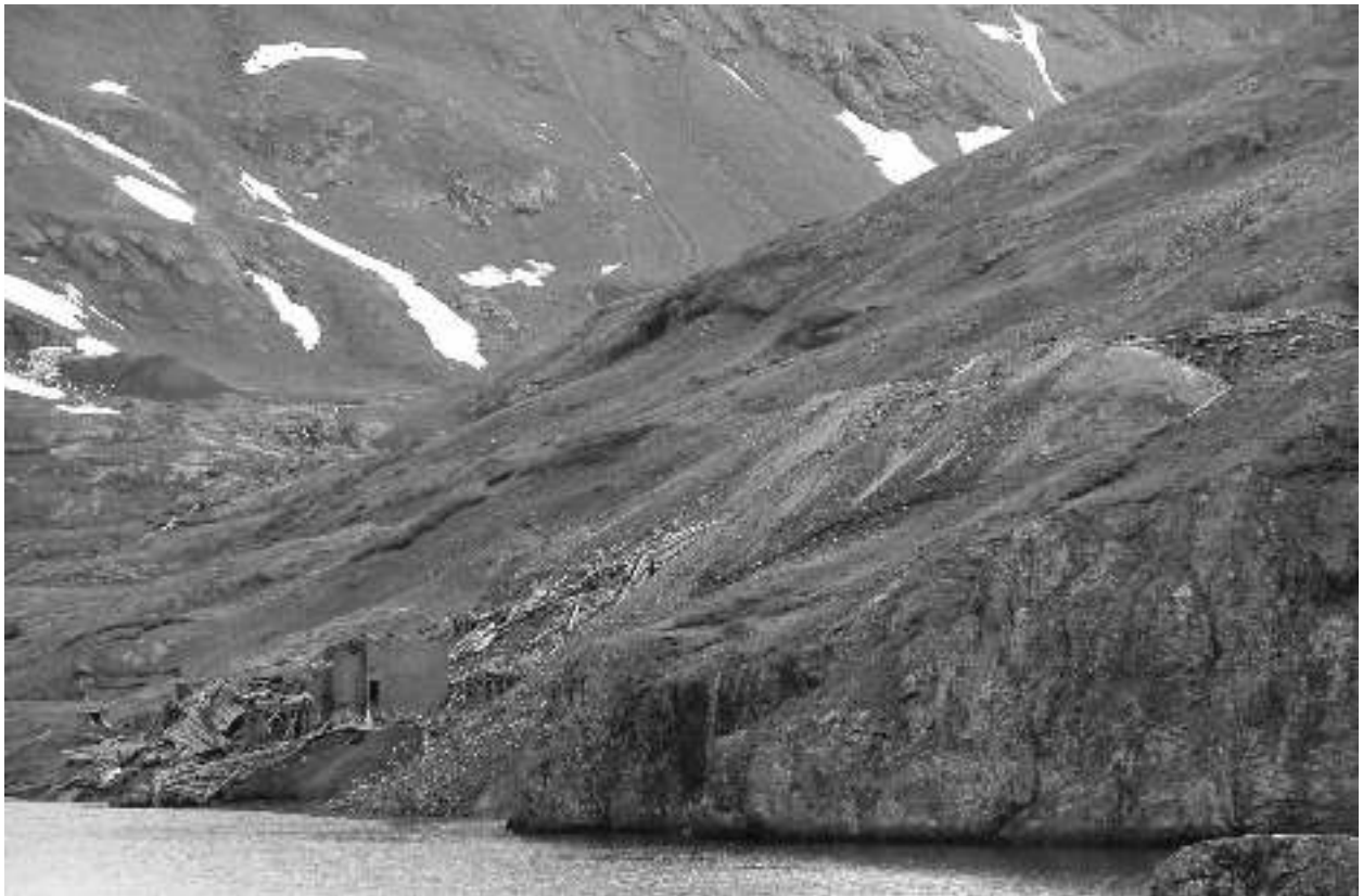
South view across Silver Lake of the remains of the Iowa Mine, August 2008. The two brick structures constituted the firewalls of the boilers inside the powerhouse, the largest building in the Iowa complex. The lower portal of the Buckeye Mine appears to sit at far left-center behind the dump. (Courtesy of Renee Vardy.)
