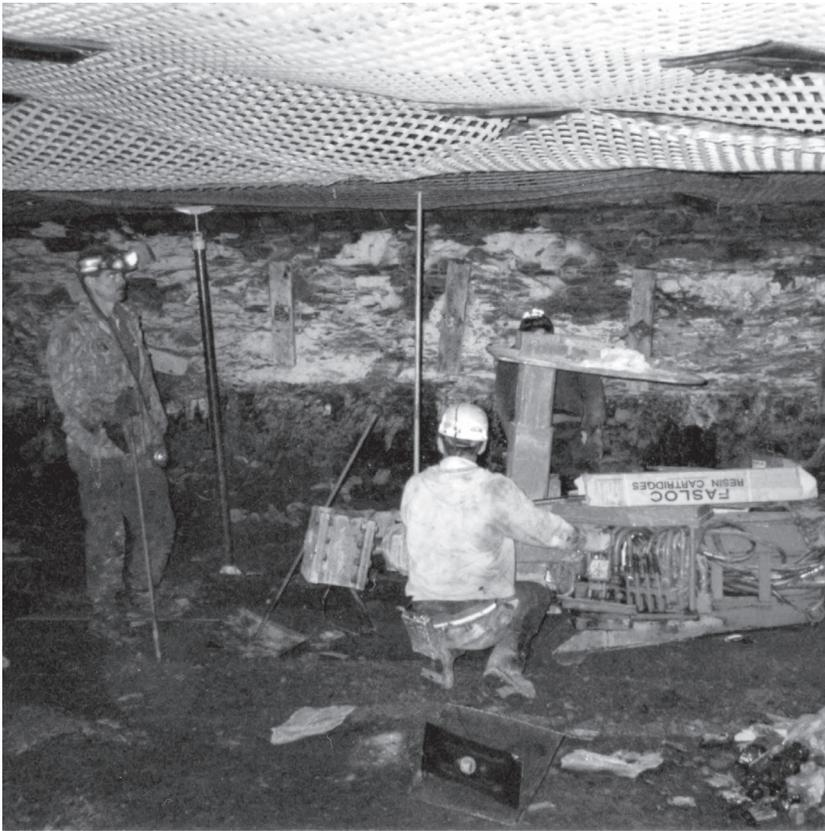
*Roof bolting and the installation of high-strength fiber mesh. (Photo courtesy of the author.)*
