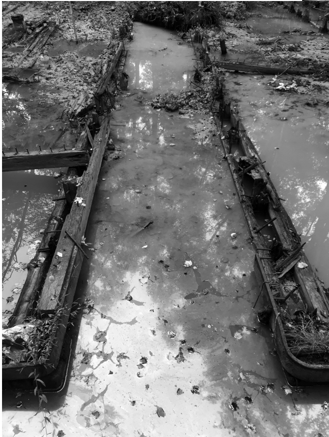
Figure 4: The central well, in which the head of the dredge once was located. All of the machin- ery was stripped from the dredge when it was abandoned after 1913. (Author's photo.)
