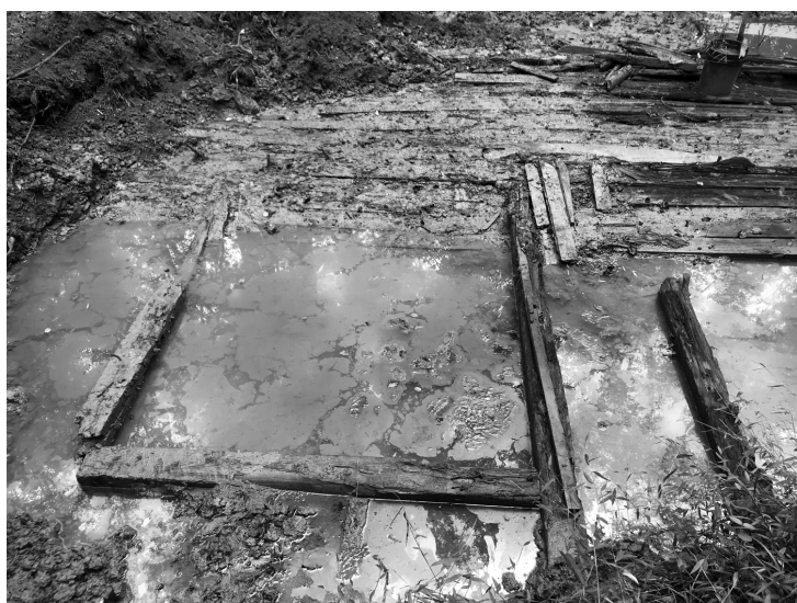
Figure 5: The toppled wall of the dredge “barn” or superstructure that once covered the machinery, on the port side. The framing outlines a doorway. (Author’s photo.)
