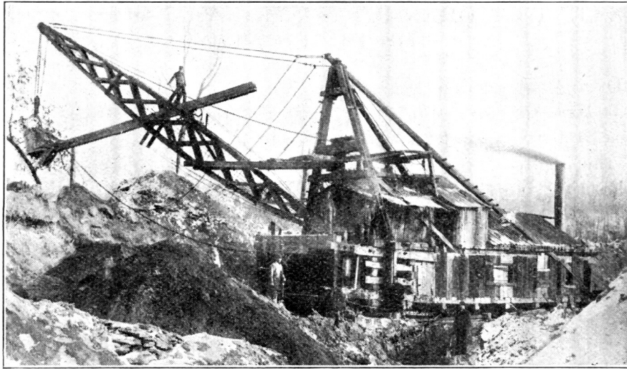
Figure 3. This homemade stripper of 1886 was made mostly of wood and was a converted dredge mounted on wheels that required a block and tackle to move. It stripped ten to fifteen feet of cover to expose a six-foot seam of coal. (From USBM Bulletin 289 (1929).)
