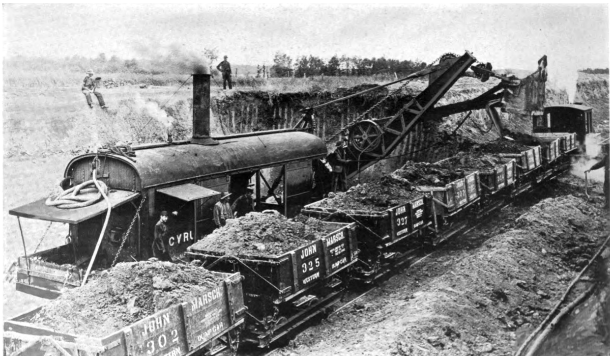
Figure 4. A steam-powered railroad shovel demonstrating almost its maximum ability to rotate. By the 1920s, these were fast being replaced by fully rotating, electric, and later diesel-powered, shovels operating on caterpillar tread. (From The Bucyrus Company (1910).)
