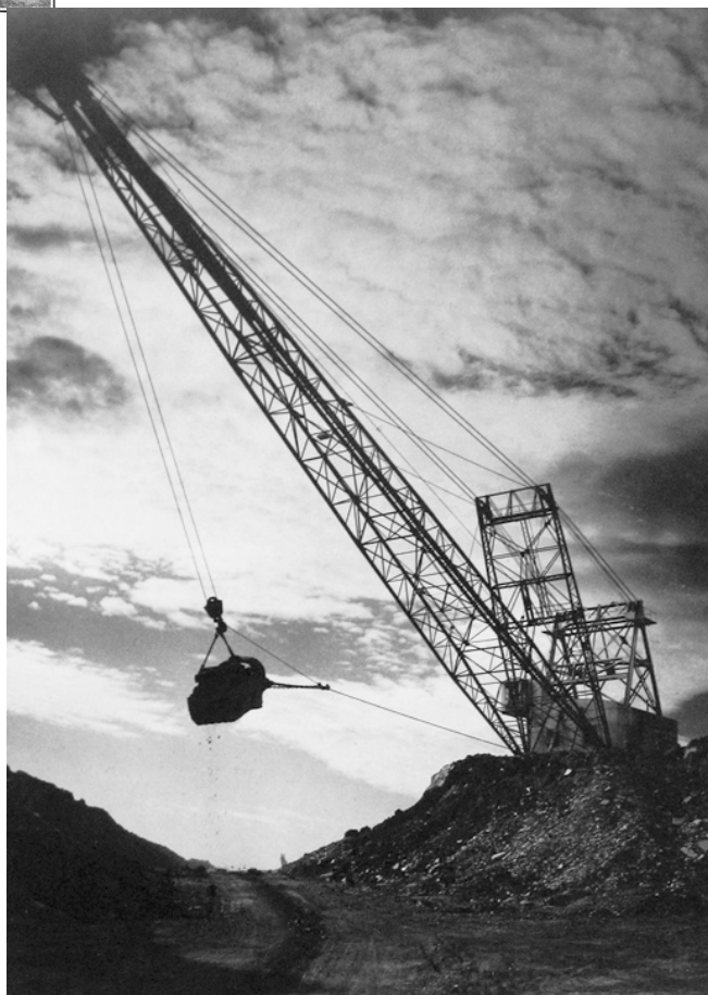
Figure 7: A dragline with a fourteen-foot bucket stripping overburden at Maumee collieries in Indiana in 1941. By World War II such equipment came with 215-foot booms allowing the mining of thin coal under heavy cover. (From William Rittase, courtesy of PDNB Gallery.)
