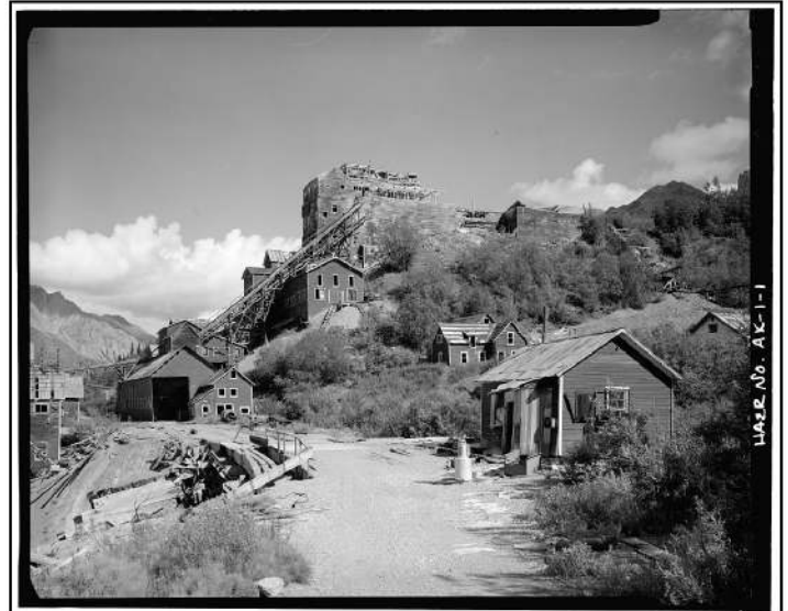
The Kennecott Mill, Alaska, viewed from the south. HAER photo by Jet Lowe, 1982. (HAER AK,20-MCAR,1--1, Library of Congress Prints and Photographs Division Washington, D.C.)
