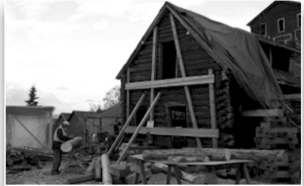
Working on the general manager's office.
