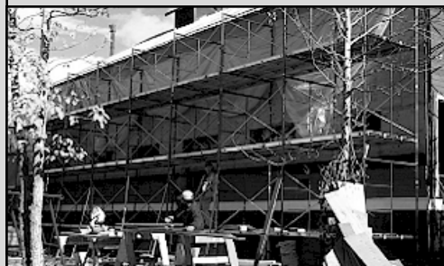
Restoring the Recreation Hall.
