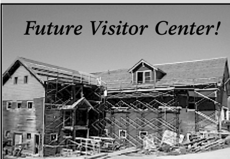
Work beginning on the Store and Post Office.
