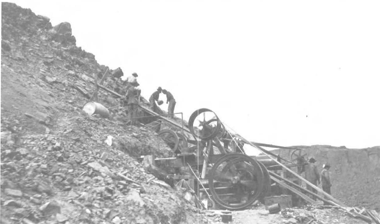
**Figure 5.** Spencer's mill operation consisted of a one cylinder gasoline engine powering a Samson Crusher with an amalgamating table. Here it is during its brief operation crushing Wingate Sandstone.
