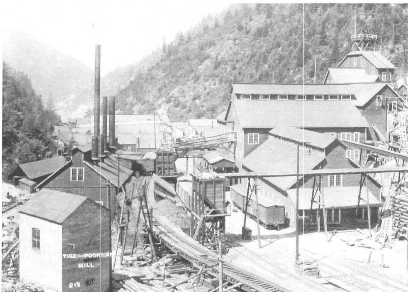
Tiger-Poorman Mine and Mill complex at Burke on Canyon Creek, Lelande Mining District, Coeur d’Alene mining region in 1904. The narrow canyon left little room for a mine and mill plant, two railroads, a wagon road, houses, offices, and businesses—forcing mine operators to build over Canyon Creek, which passes through an underground conduit. (Photo 8 -X219, Barnard-Stockbridge Collection, University of Idaho Library.)
