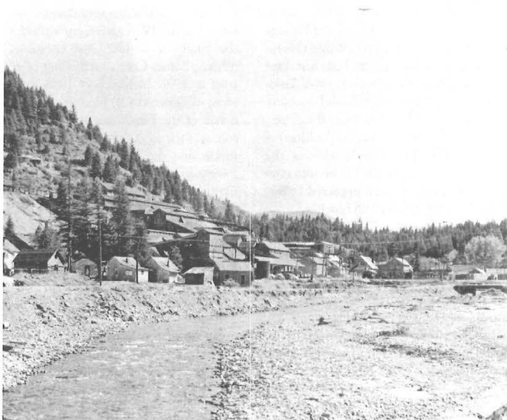
Morning Mill on the South Fork of the Coeur d'Alene River near Mullan, 1904 (by F.L. Ransome) and 1951 (by R.E. Wallace). In 1904, the river channel was choked with coarse jig tailings. In 1951, long after all of the mills had converted to flotation, all tailings have been washed further downstream. (U.S. Geological Survey Photographic Collection, Denver, Colorado).
