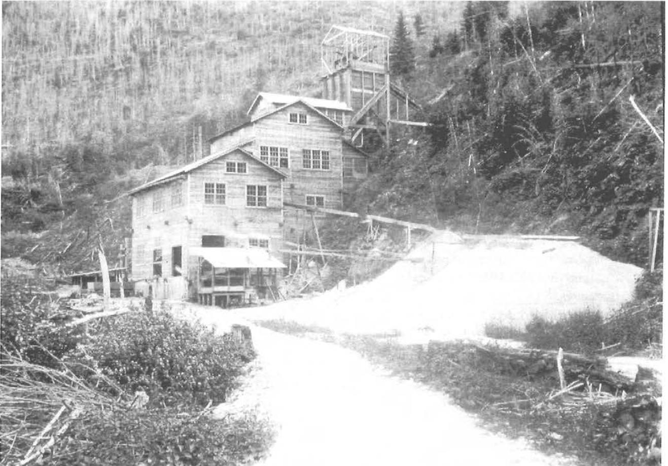
Mill of the Big Creek Mining Co., Big Creek, Yreka Mining District, Coeur d'Alene mining region, 1920. This mill sent tailings into Big Creek immediately above the intake for the town of Kellogg's water system. Promptly restrained by court order, the company built a flume which took its tailings around the water intake. The stockpiles may be concentrates. (Photo 8-X607A, Barnard-Stockbridge Collection, University of Idaho Library.)
