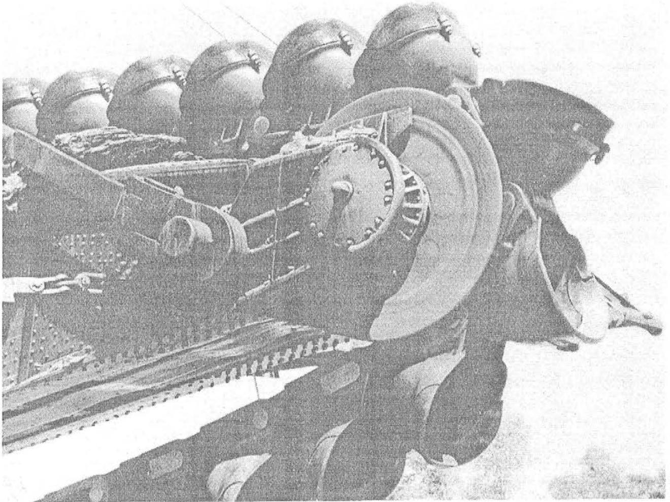
Figure 3 Lower end of digging ladder with 18 cubic foot buckets. Showing lower tumbler arrangement, buckets with bolted on lips, and part of ladder suspension. From *Yuba Placer Mining Dredges*, Yuba Manufacturing Co., San Francisco, 1952.
