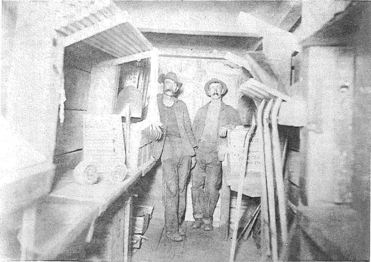
A powder magazine on the 600' level of the Spray mine. Loading sticks used to tamp the dynamite in the drilled holes are in the upper left while rolls of fire fuse and boxes of blasting caps are below. The miner on the right is leaning on fifty-pound boxes of Hercules dynamite. Courtesy of the Bisbee Mining & Historical Museum.
