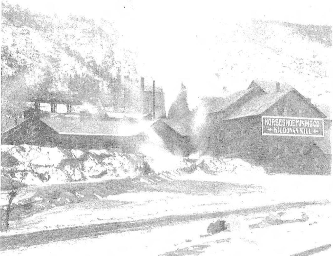
The Horseshoe Mining Co. constructed The Kildonan Mill in 1895. Originally designed to use the chlorination process, it was later modified for cyanide. The plant operated intermittently until damaged by fire in 1912.
